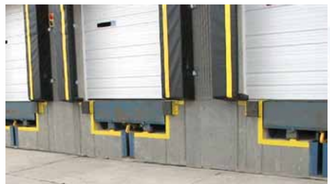
The PIT-HOOK™ vehicle restraint, as installed in this warehouse, is a non-impact design that allows unobstructed access for snow removal, smaller delivery trucks and trucks with tail gates.
